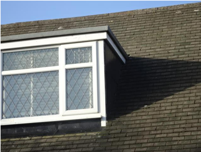
Roof and dormer window
