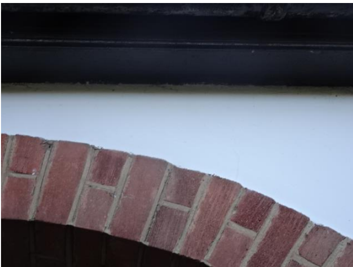
Wall top - sealed
